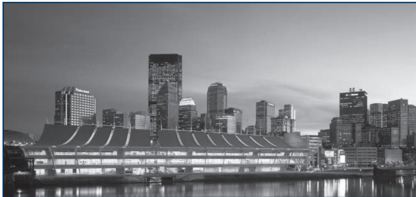
Located in the heart of downtown Pittsburgh, the stunning new $354 million David L. Lawrence Convention Center graces the banks of the Allegheny River. It is the first certified "green" convention center in the United States. Photo courtesy of the Greater Pittsburgh Convention and Visitor's Bureau.
